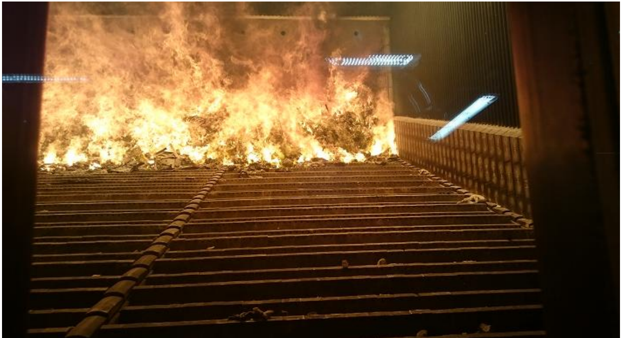
First combustion of waste on Line 1, viewed from the boiler's viewport (Copyright PML)
